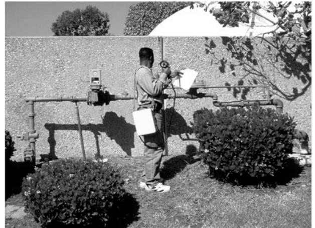
Fig. 2 Photograph showing man checking a gas meter for leaks with a hand-carried detection unit.
