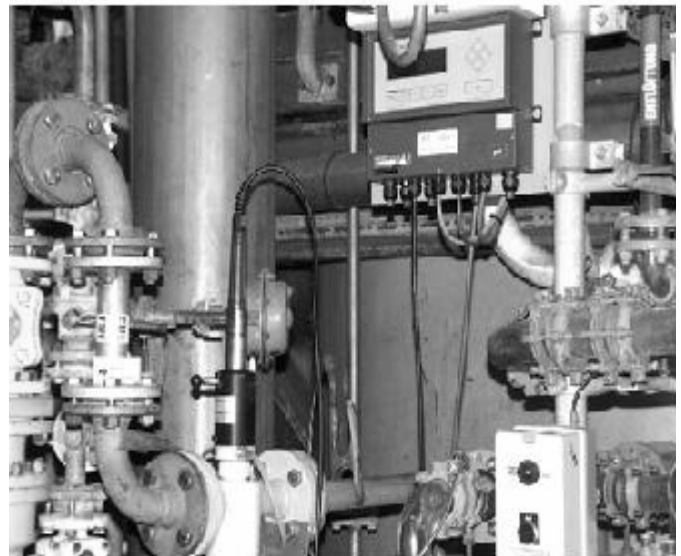
Fig.7 Picture showing image transmitted after the gas leakage detection
